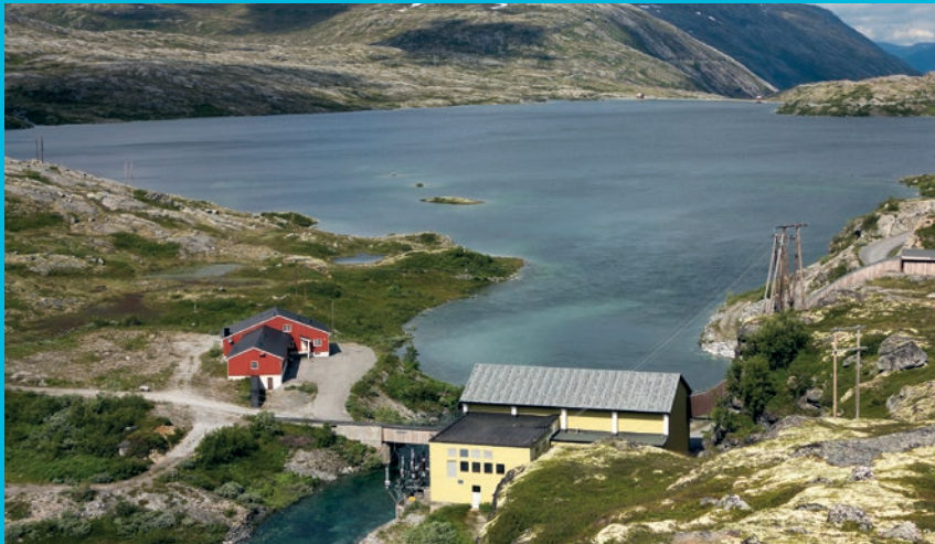
Osbu power station
