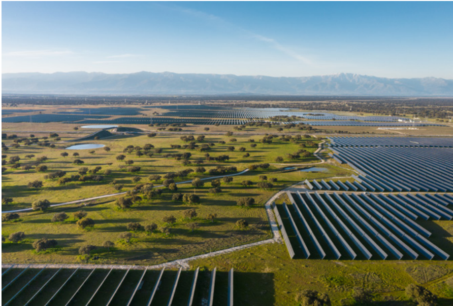
Location: Talayuela Solar Plant, Spain
